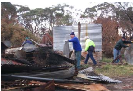
Members removing fire damaged materials
